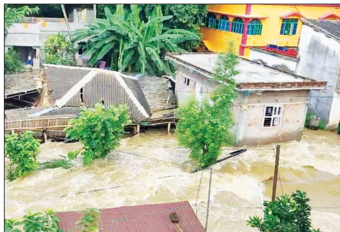
Figure 16 : Buildings submerged due to floods in West Bengal/ Source: Wire _ 26/09/2024 (Media)
