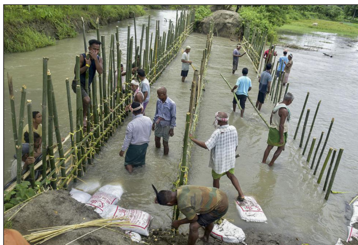
Figure 3: Villagers repaying the embankment breach caused due to flood in Assam| Source : The Hindu_21/07/2024 (Media)
