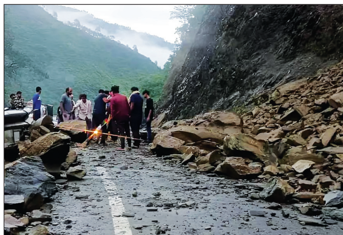
Figure 14 : Road Blocked in Chamoli district | Source: The Indian Express _ 11-08-2024 (Media)
