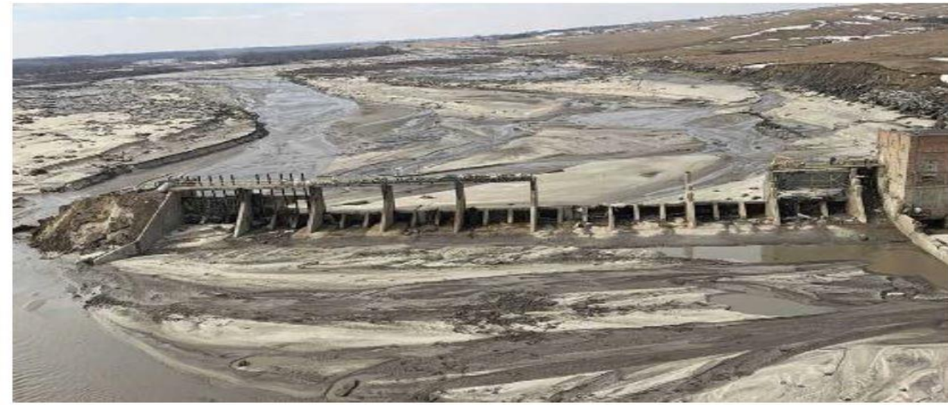
Spencer Dam, USA – Gate operational problem due to ice
