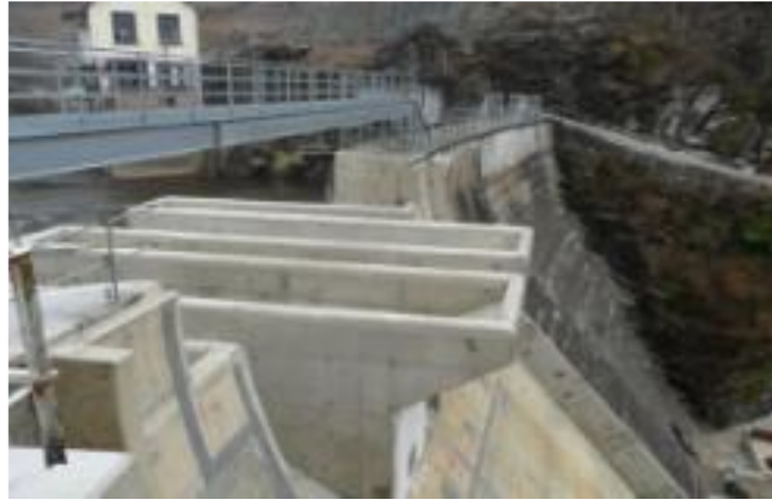
Key Weir types with overhang and without them.
