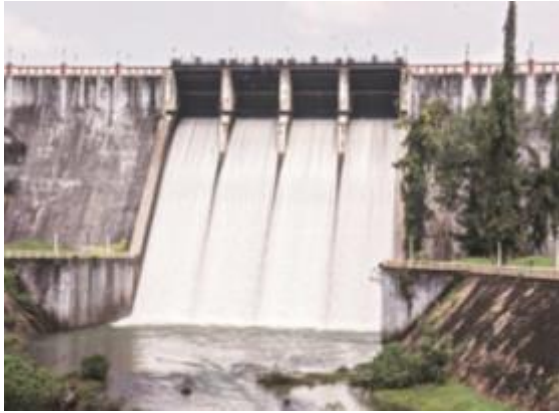
Service spillway, Controlled ogee crest
