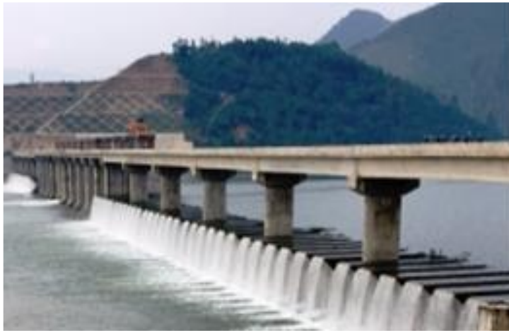
Piano Key Weir – Van Phnong Dam, Vietnam
