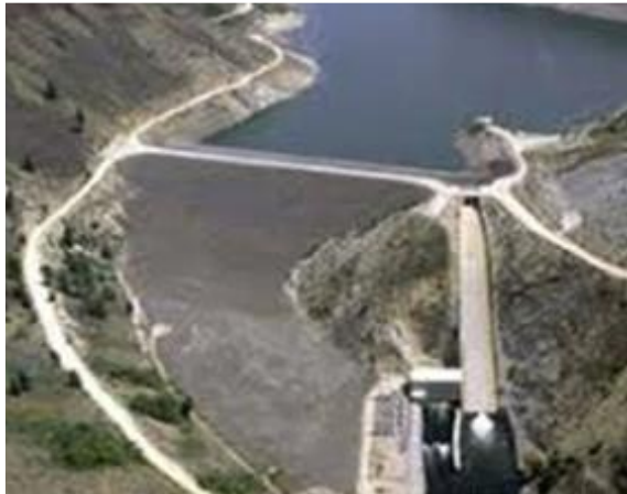
Service spillway, on left abutment of an embankment dam
