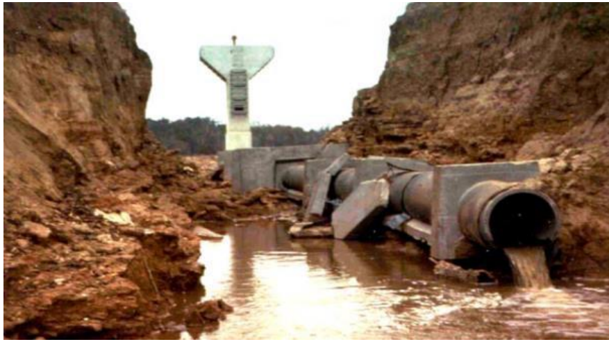
Internal erosion around conduit in embankment dam
