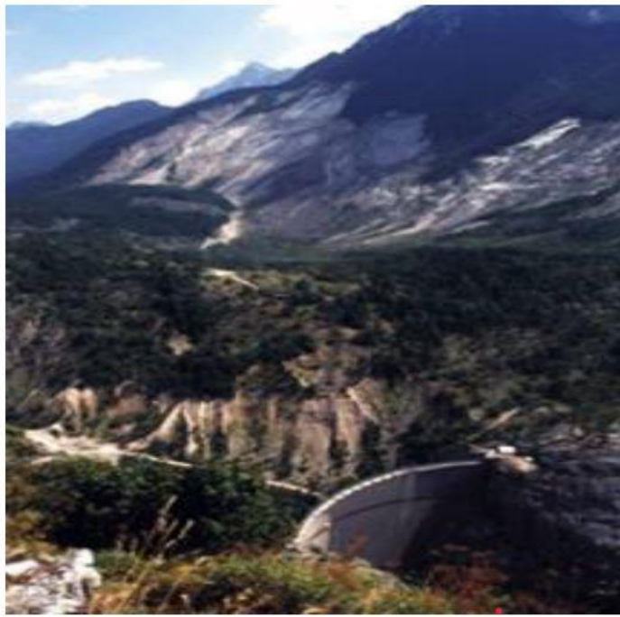
Vajont Dam, Italy – Left bank sliding
