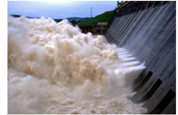
Typical bottom outlet in overflow dam section
