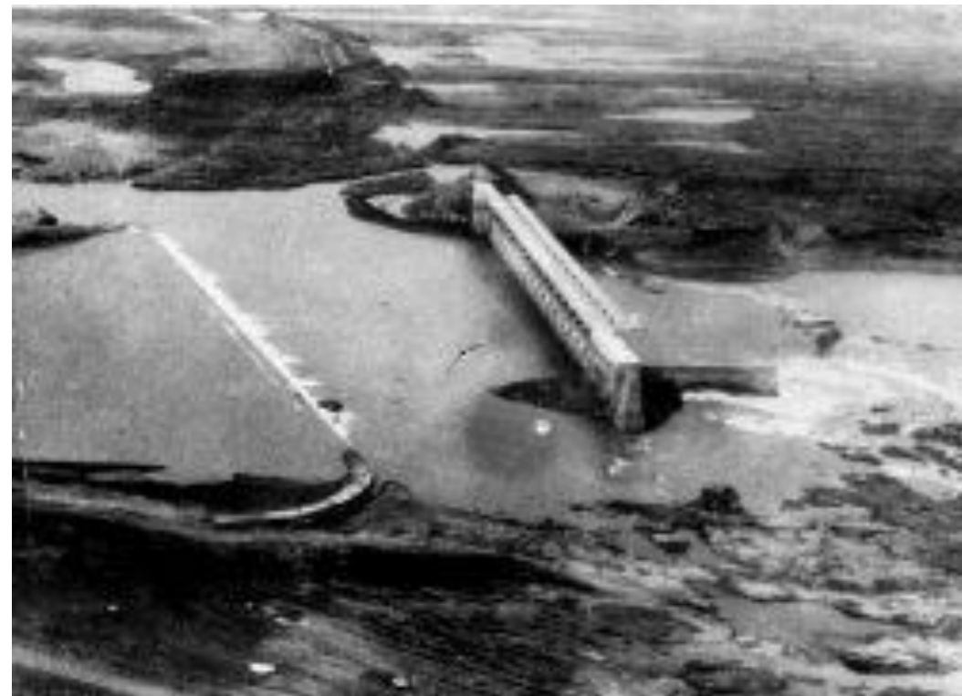
Machhu dam disaster of 1979 in Gujarat
