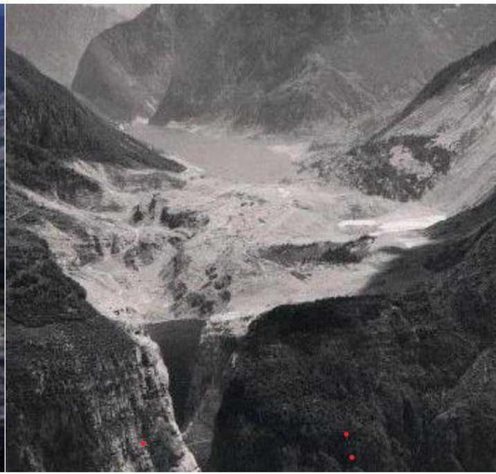
Vajont Dam, Italy – Left bank sliding
