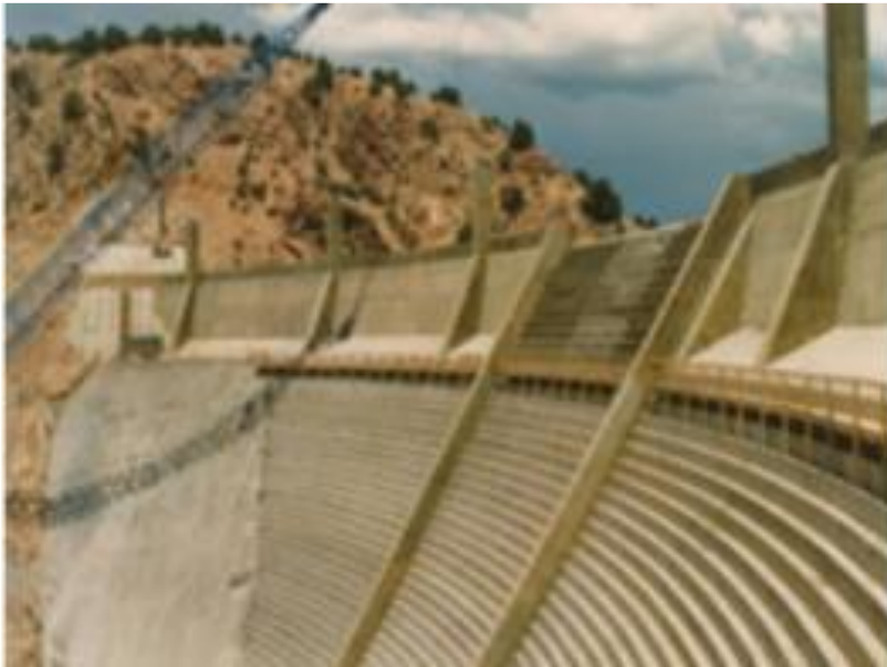
Concrete overtopping protection for Santa Cruz Dam
