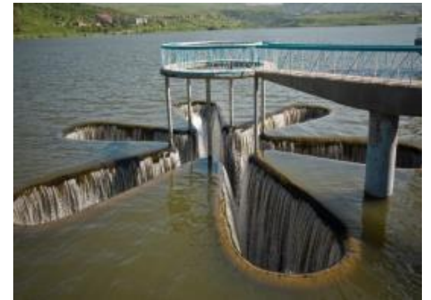
Service spillway, Control structure - Morning glory and special weir
