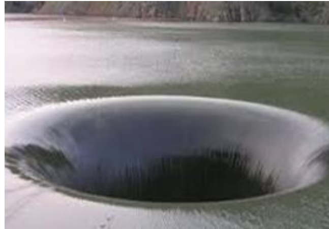
Service spillway, Control structure - Morning glory and special weir
