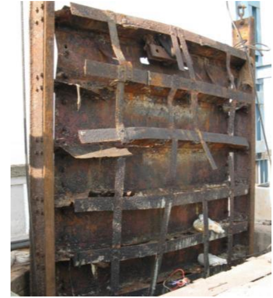
Condition of sluice gates in 2018
