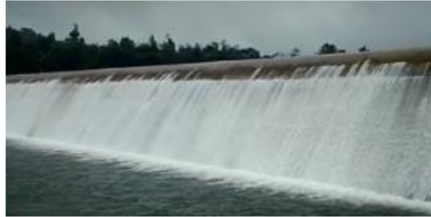
Service spillway, uncontrolled
