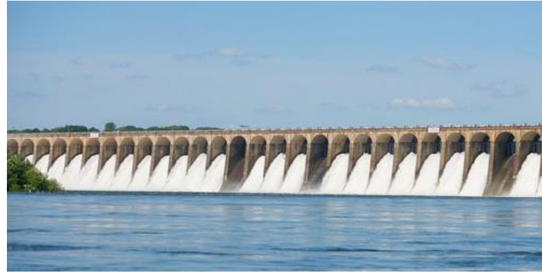
Wilson Dam, Alabama. Orifice spillway
