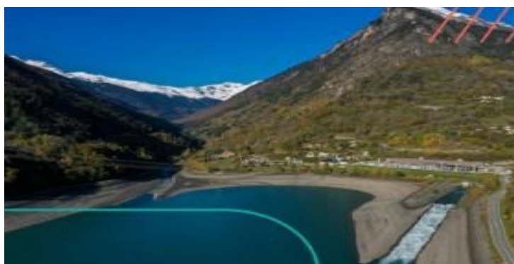
Figure A1.11: Grand Maison hydropower project
