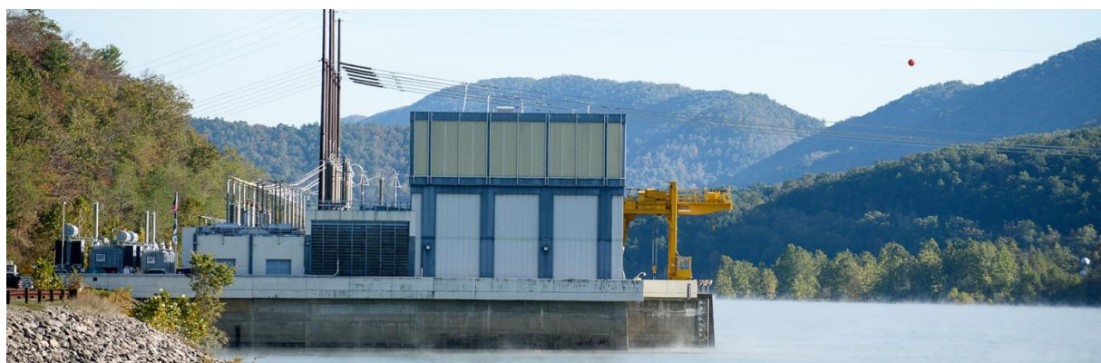
Figure A1.1: Bath County Pumped Storage Station
