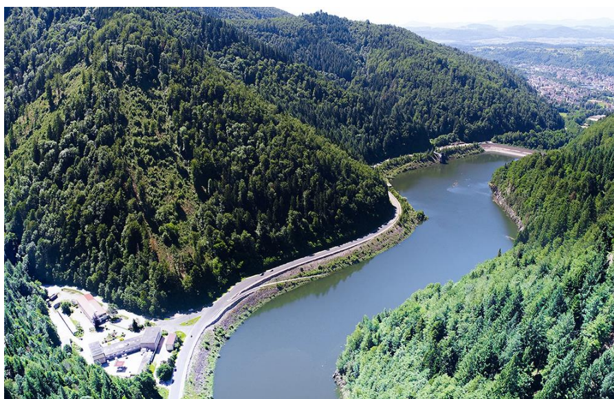
Figure A1.6: Wehr Pumped Storage Power Plant
