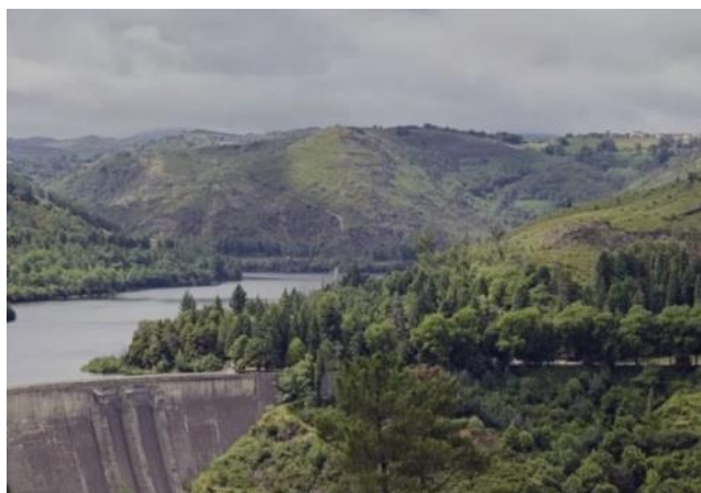
Figure A1.7 Frades II PSP project in Portugal
