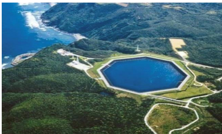
Okinawa PSP facility that use Philippine sea water at Okinawa Island in Japan
