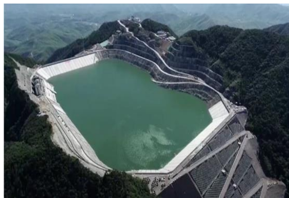
Upper Reservoir of Changlongshan PSP
