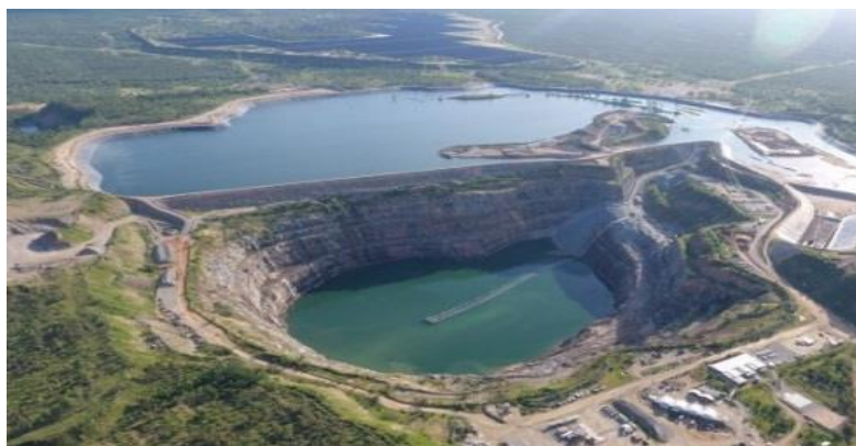
Figure A1.10: Kidston Gold Mine's upper and lower pits.to be used as Reservoirs for PSP
