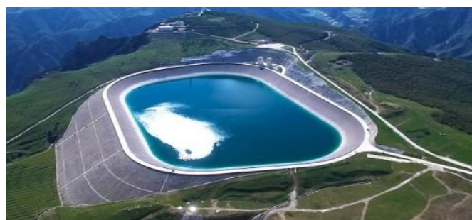
Hohhot PSP Plant in China (1,224MW)
