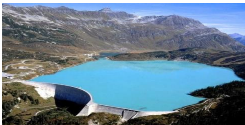
Figure A1.8 Upper reservoir for Kops II PSP
