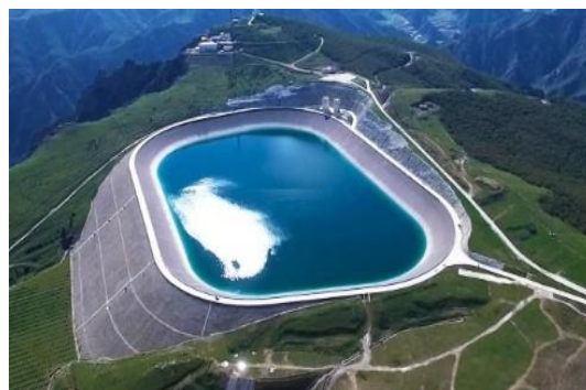
Upper Reservoir of Hohhot PSP
