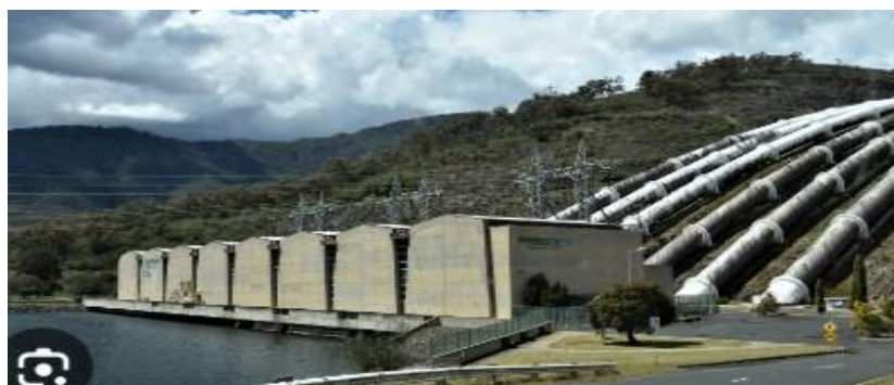
Figure A1.3: Tumut 3 Pumped Hydro Power Station
