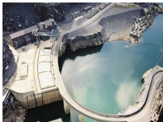
Dinorwig PSP in Abandoned mine. UK
