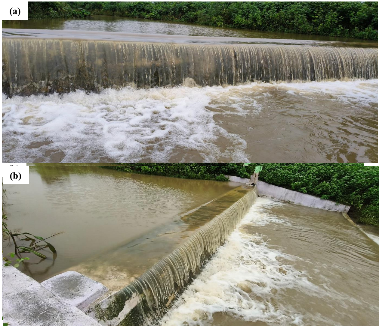
Fig. 6: Check dam in Telangana. (Source: National Water Mission, Ministry of Jal Shakti, Department of Water Resources, RD & GR, Government of India).
