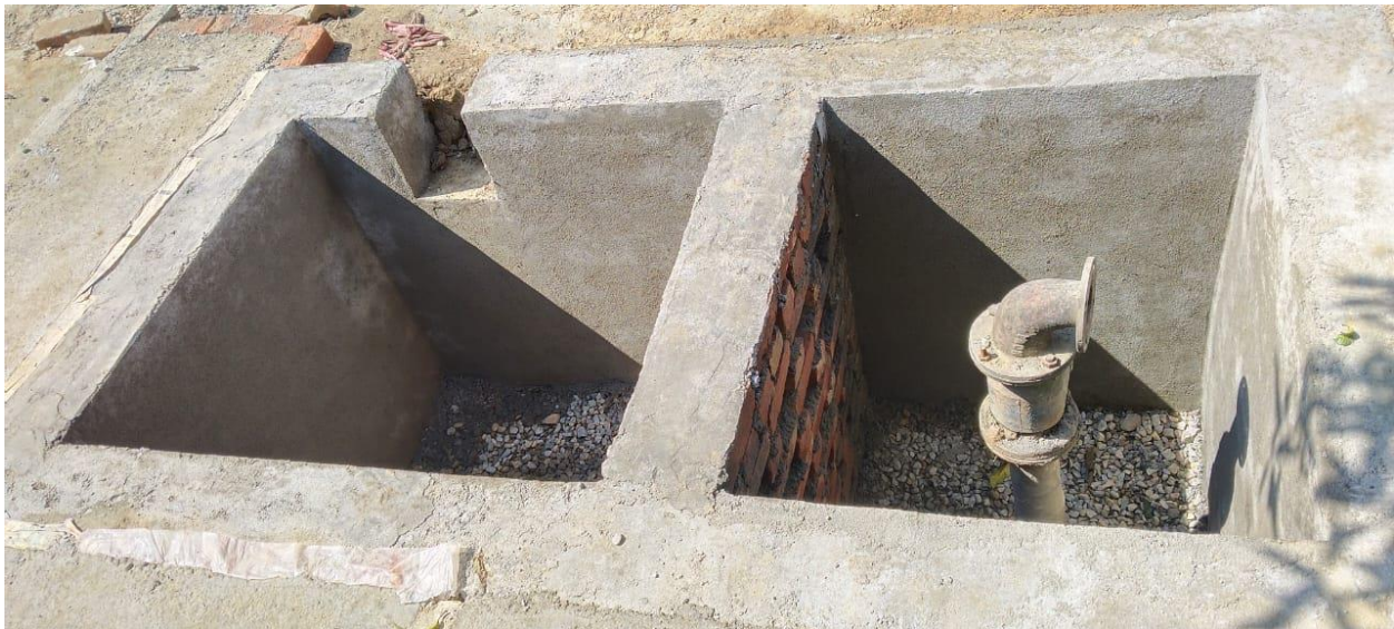
Fig. 2: Groundwater recharge structure constructed in Udham Singh Nagar. (Source: National Water Mission, Ministry of Jal Shakti, Department of Water Resources, RD & GR, Government of India).
