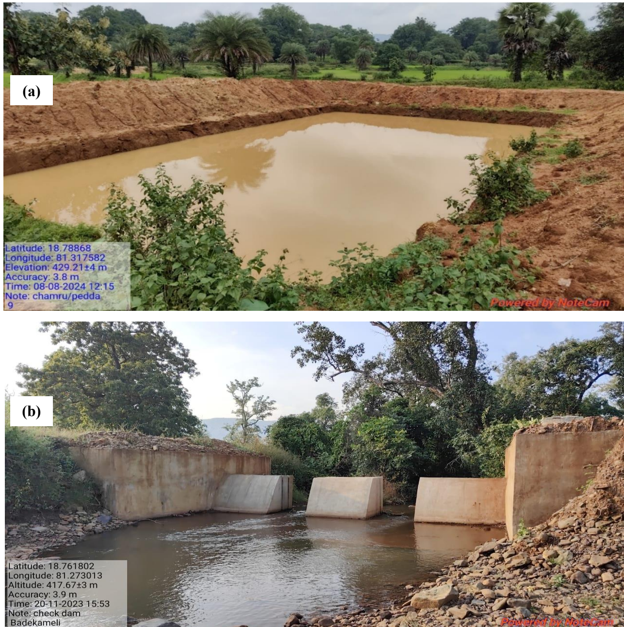
Fig. 9: Water conservation structures: (a) Farm pond in Gamawada and (b) Check dam in Badekameli. (Source: National Water Mission, Ministry of Jal Shakti, Department of Water Resources, RD & GR, Government of India).
