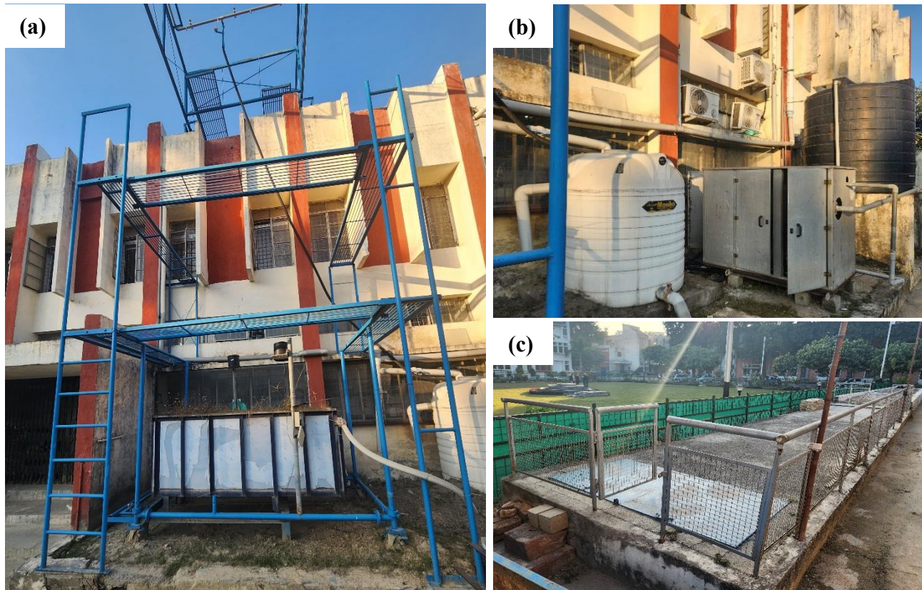
Fig. 1: Rooftop rainwater harvesting system installed at the Department of Water Resources Development & Management, IIT Roorkee. The system utilizes a combination of recharge pits and recharge shafts for effective groundwater recharge, as illustrated in images (a), (b), and (c).
